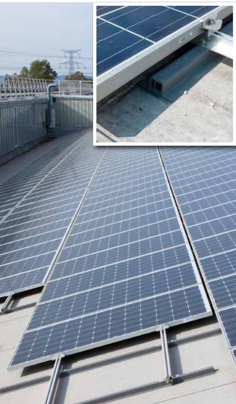
Industrial building Valéo – France 24,500 m 2 RENOLIT ALKORPLAN F + RENOLIT ALKORPLAN Solar profiles
