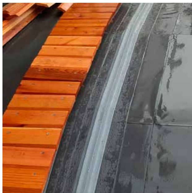
Wooden slats are secured to RENOLIT ALKORPLAN Solar profiles.
