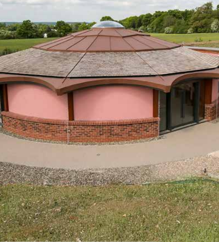
Cemetery prayer room – United Kingdom RENOLIT ALKORPLAN Solar profiles as basis for wooden tiles
