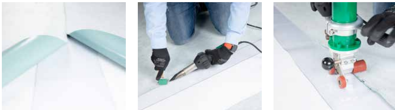
Welding sealing for longitudinal overlap.
