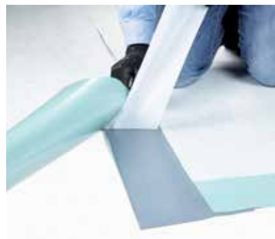
Butyl tape sealing for transversal overlap.
